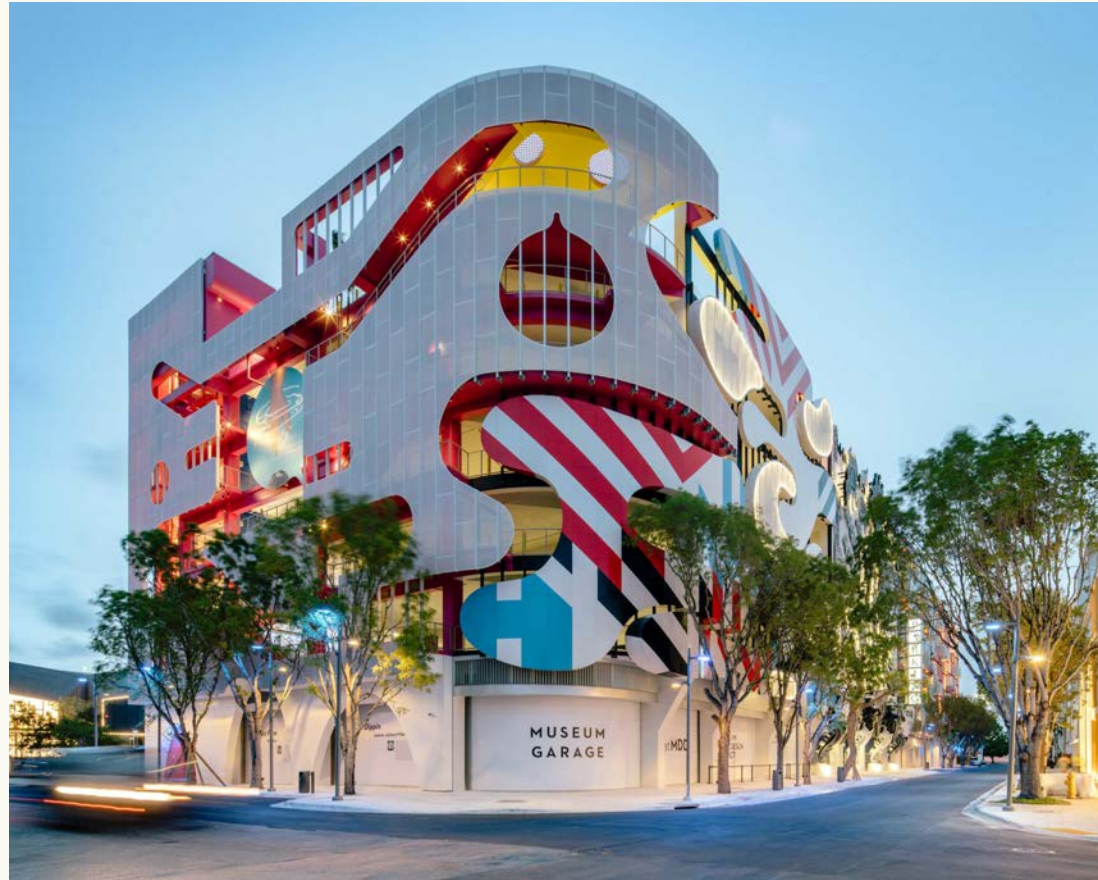
Museum Garage, photographed by Imagen Subliminal in Miami, FL. The lead architect was Terence Riley- but he selected WORKac, J. Mayer H., Clavel Arquitectos, and Nicolas Buffe to also work on facades.
